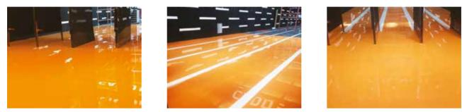
It is the most suitable system in terms of safety procedures. The surface can be cleaned easily as it has no joints. Upon request the color can be changed by applying topcoat paint.
